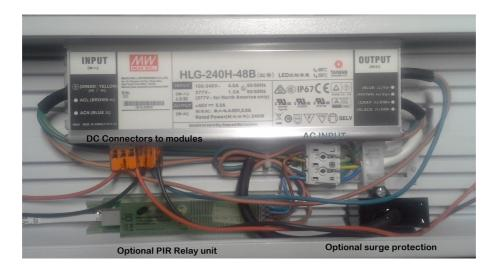
Power cable entry is from the rear of the Luminaire via the cable gland.
